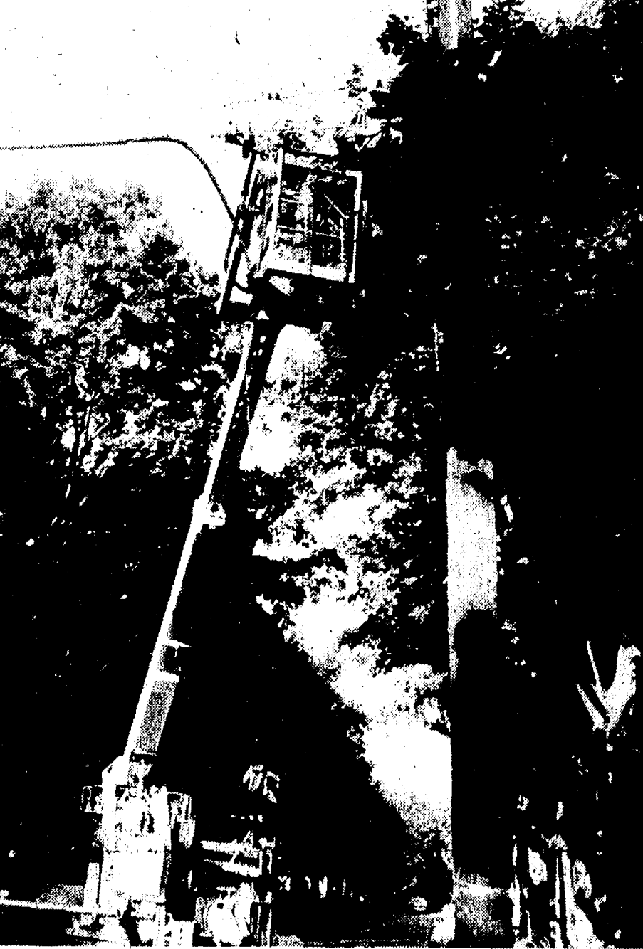
WIRES MOVED: Telephone and electric wires stretching across W. Middle St. had to be dropped to street level during yesterday's house-moving. There was no interruption in service. Here, a telephone company crew detaches a cable from a utility pole.
