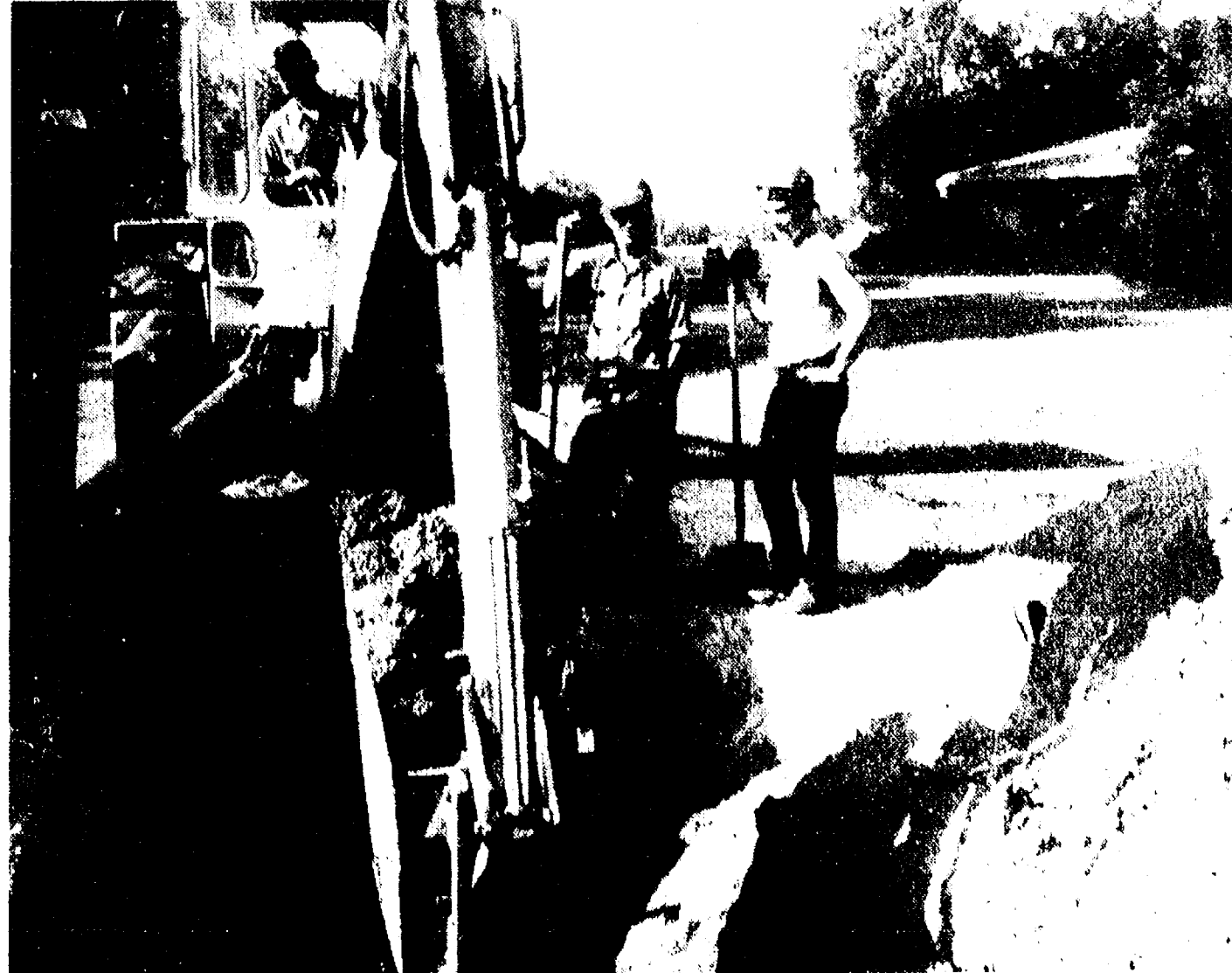
WATER MAIN EXTENDED: Village workers are putting in a new water main along Freer Rd. south from Washington St. In photo are Ellsworth
